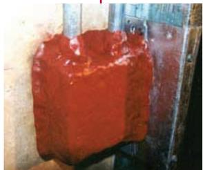
Externally applied to switch and receptacle boxes, pads are UL tested and Classified to permit larger boxes and reduced spacing in gypsum board walls.
