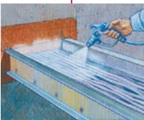
Water-based, spray-applied coating used to provide short term circuit integrity and improved flame spread characteristics for grouped electrical cables.
