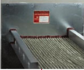
Lightweight, easily fabricated panels surface mount to walls and floors to provide a neat, clean firestop seal for medium to large openings with a variety of penetrants in fire-rated floors and walls.
