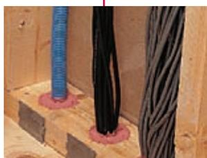
BlazeStop™ Series WF300 Firestop Caulk is designed for use in sealing through-penetrations and gaps in fire resistance-rated wood frame construction.
